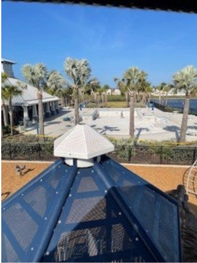
View of pool work construction from the playground structure.
